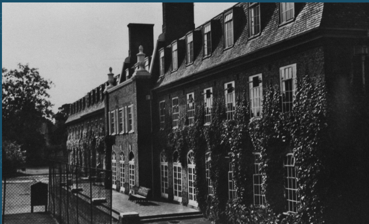
Bexley nurses' accommodation block at the old Bexley Mental Hospital.
